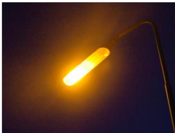
**Figure 3.10:** A low pressure sodium streetlamp.
